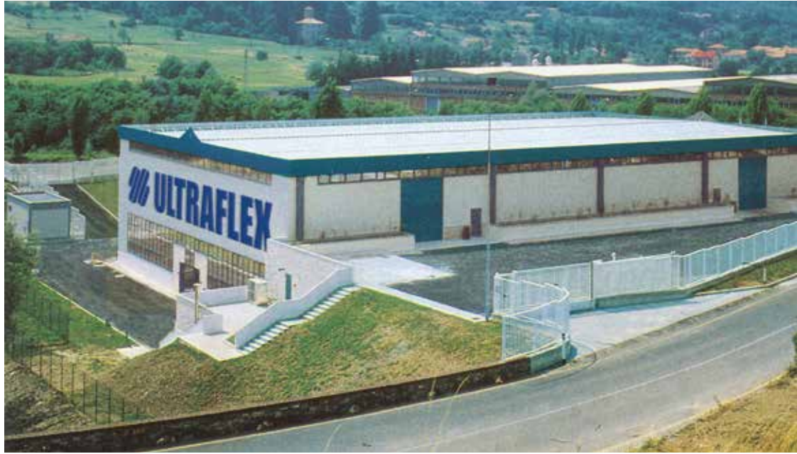
ULTRAFLEX - Factory in Casella
