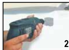
2 Attach the flange at the point you want to place the light and open the holes using a drill
