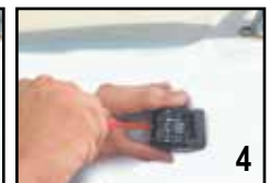
4 Screw until the rawl plugs are secured
