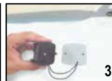
3 Pass the wires through the lower hole and fit the light's rawl plugs in the side holes
